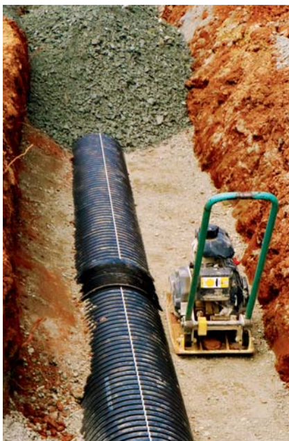
SIROPLAST-K multi-purpose pipes for combined discharge of drainage and surface water
