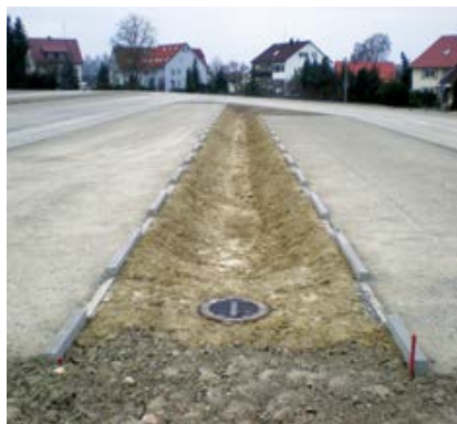
Parking area with swale infiltration
