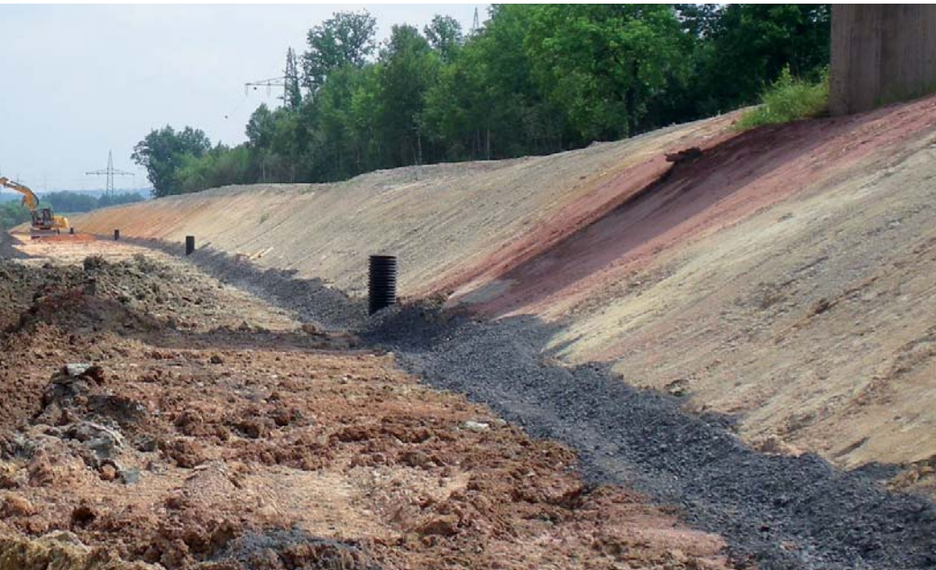
Inlet chamber in trough with small laying depth
