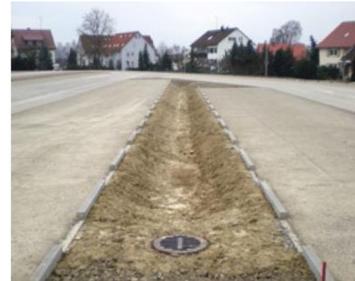
Car park with drainage swale and open curb on both sides
