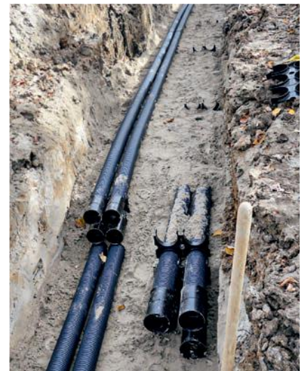
Subsoil HEKAPLUS cable ducts for large-scale connection of solar modules
