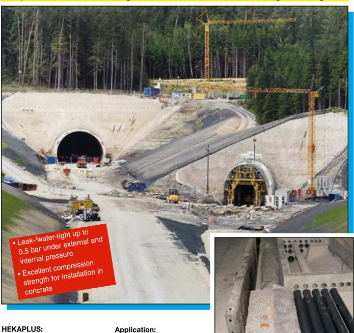
PE-HD ducting system in twin wall design for projects in the field of infrastructure and construction engineering where special requirements have to be met. HEKAPLUS is produced in accordance with DIN 16961 and meets the increased requirements of EN 61386-24.
