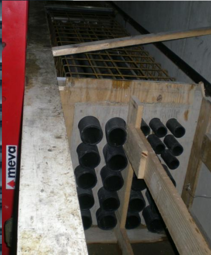
Casing to cable chute
