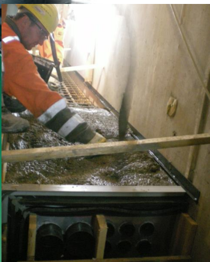
Placing of concrete and allow filling between pipe intervals
