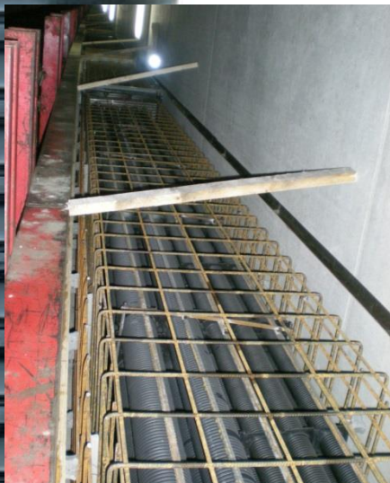
Duct package in armoring
