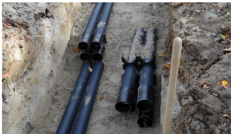
Multi-strand installation of HEKAPLAST-S in packages with spacers
