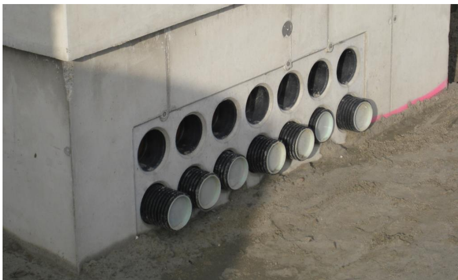
Professional connection to distribution manhole
