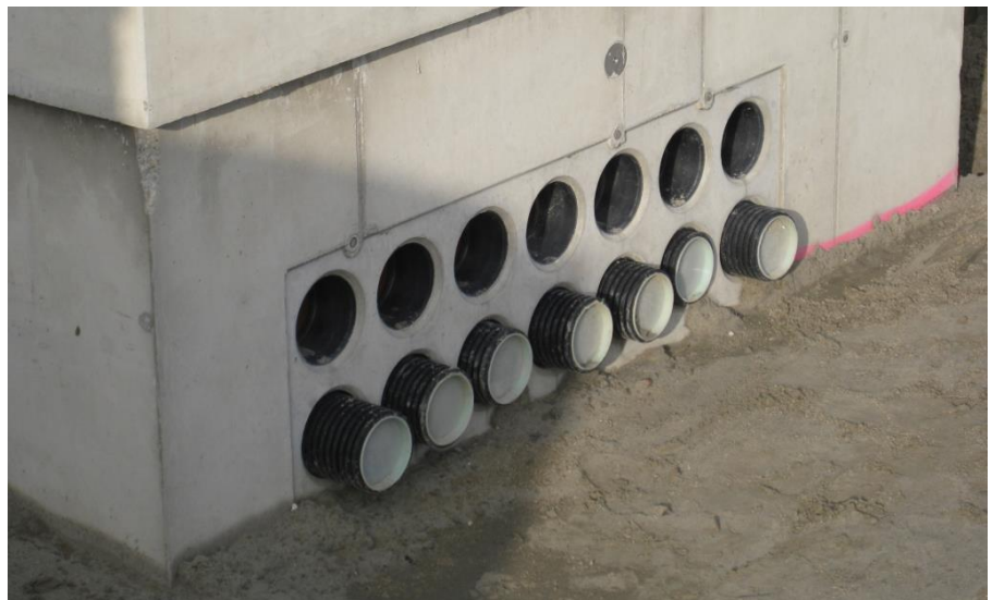
Professional connection to distribution manhole
