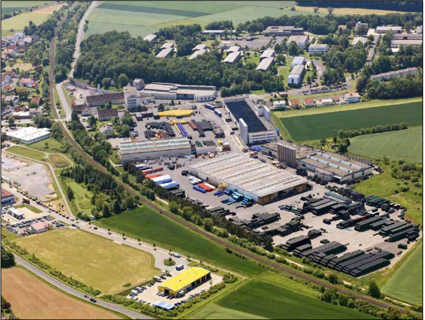
Head office and Oerlenbach plant
