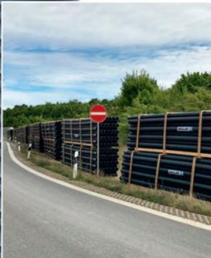
Professional site storage of civil engineering drainage pipes SIROPLAST-K DN150 at rest area Kreuzfeld-West
