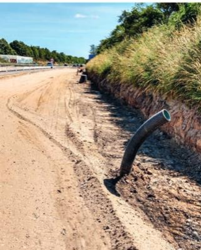
Connection of swale drainage with flexible pipe line AQUATUB-RwR DN 150
