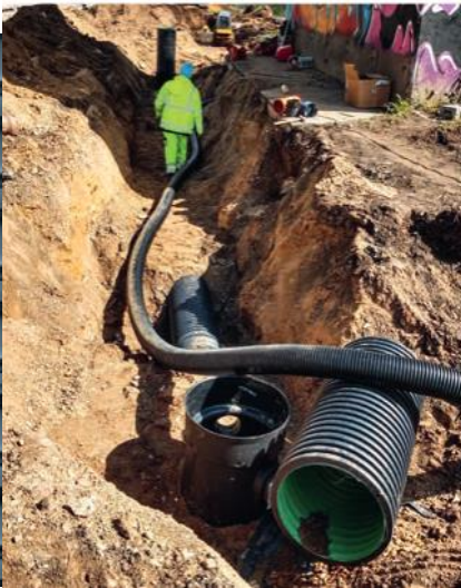
Chamber system MULTI-inspect DUO with carrier pipe AQUATUB-Rw in confined space
