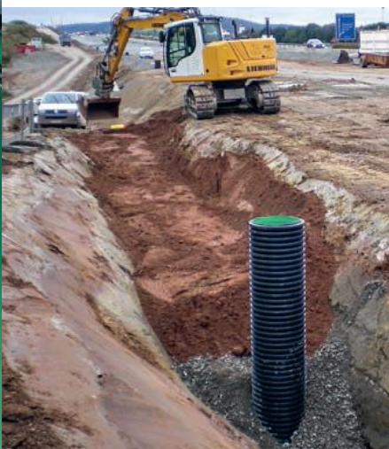
Exit Geiselwind: drainage of access road with MULTI-inspect 600
