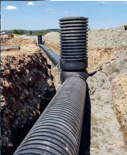
Carrier line AQUATUB-Rw in combination with MULTI-inspect 600 chamber system
